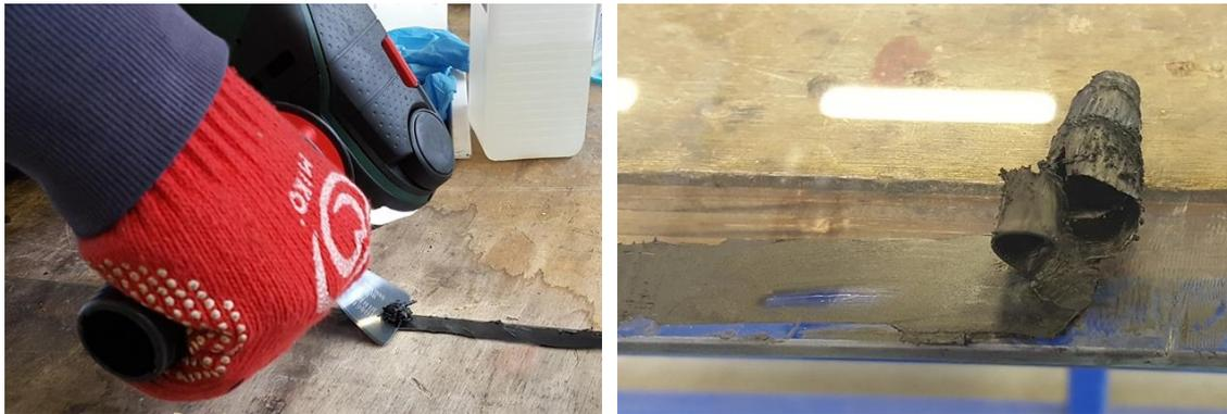
*Figure 2: Removal of PIB/Silicone from glass edge with vibrating scraper.*
