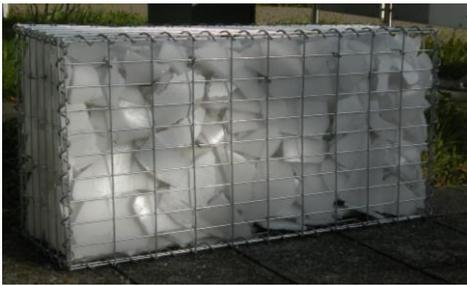
**Picture 12:** Gabione bench filled with used quartz crucibles pieces
